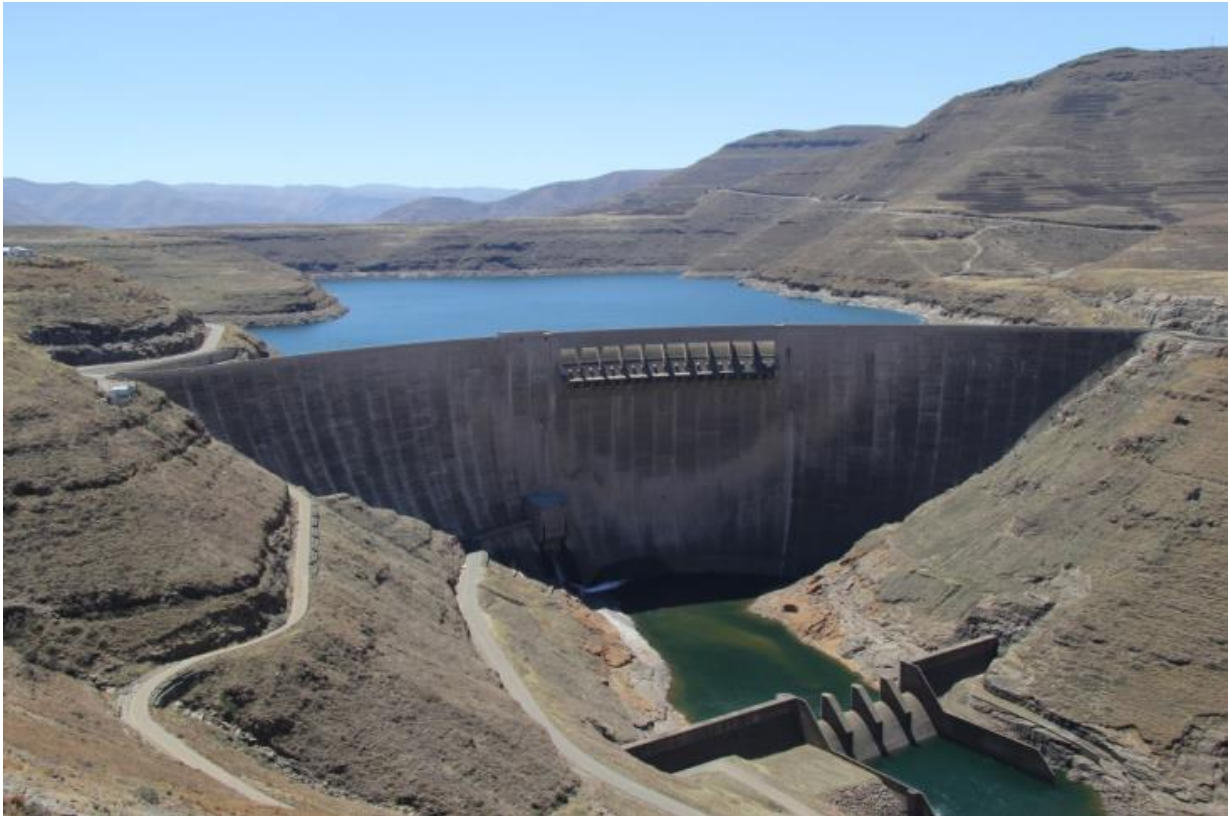
Figure 2. The Katse Dam wall.
