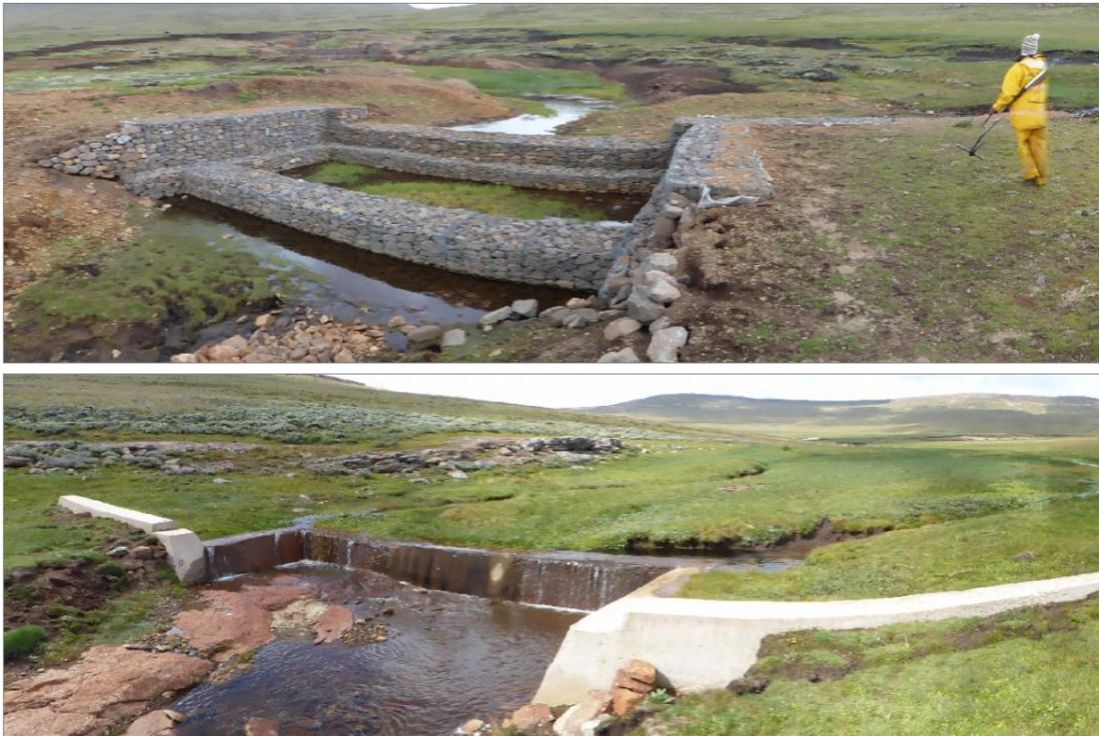
Figure 31. Rock gabions and concrete structures used in restoration efforts in Katse wetlands. Note the lack of water retention behind the rock gabion compared with the concrete structure.
