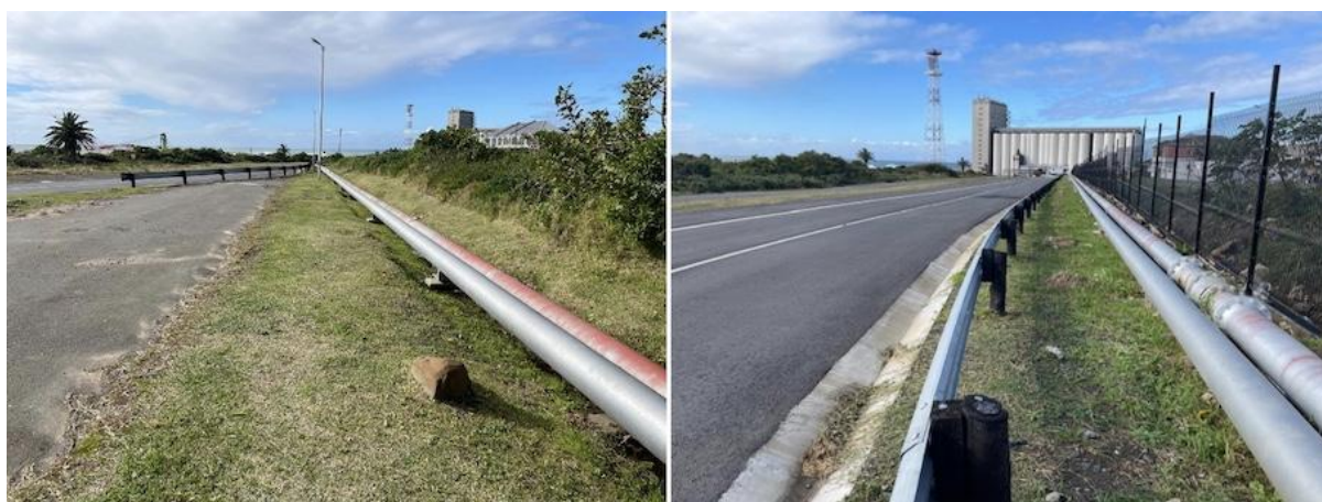
Plate 2: Views east along the proposed marine outfall pipeline route (Photos: J Kaplan).
