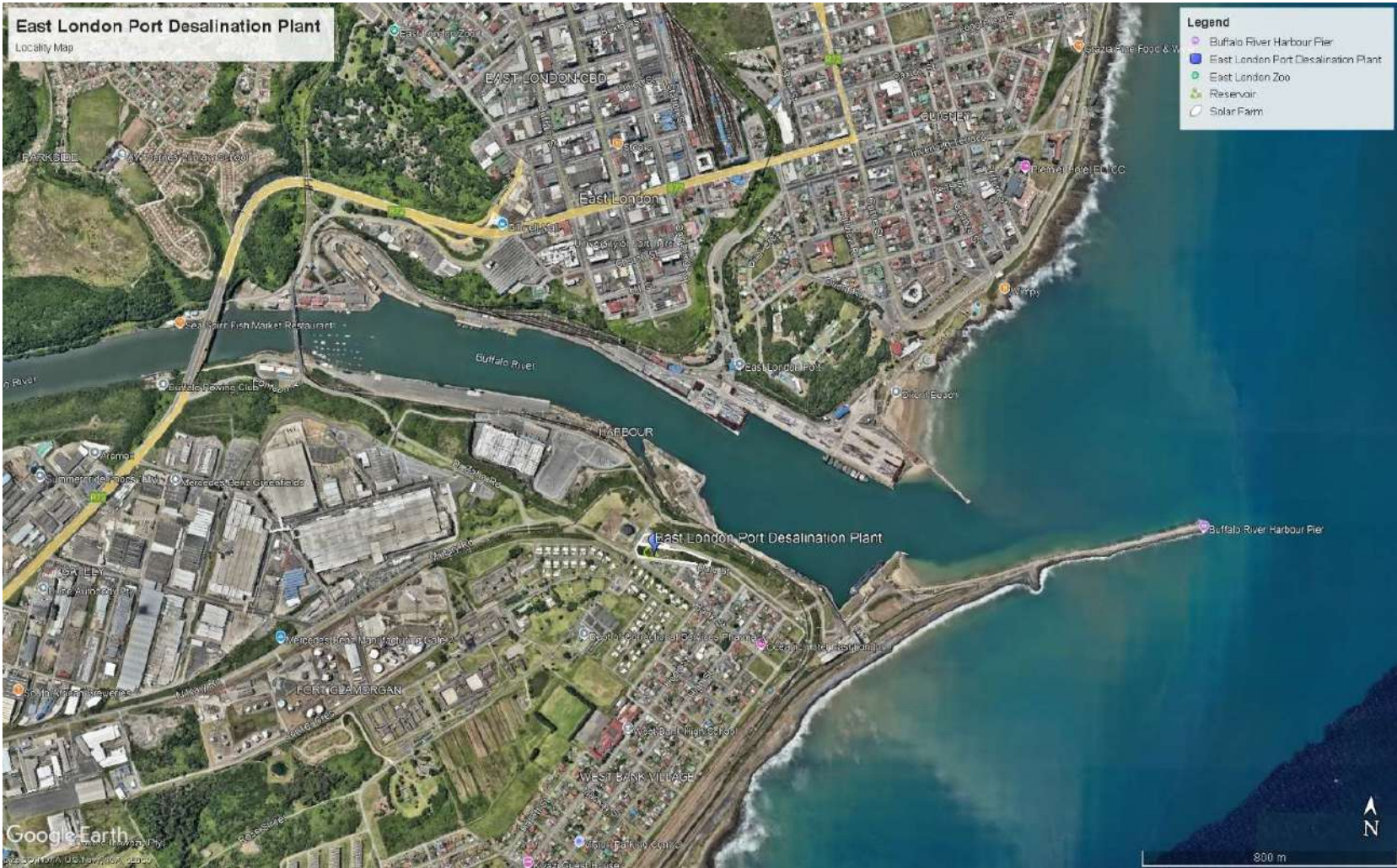
Figure 1: Regional locality of the desalination plant.
