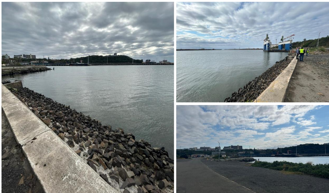
Figure 3.21. The EFZ of the proposed intake site (site visit photos taken in August 2025).
