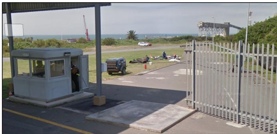
Figure 8.1. Google Streetview image of the proposed RO Plant site (grassed area between the tar roads to the left of screen).
