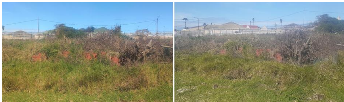
Figure 8.21. Examples of the remains of the demolished houses on the proposed PV site. The red brick walling visible in the images is typical of much 1930's South African residential housing (Source: Anchor Environmental).
