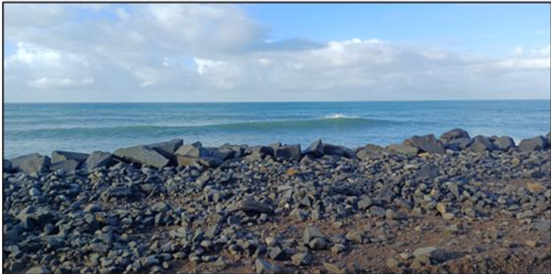
Figure 8.7. The beach to the south of the Port of East London entrance is comprised almost entirely of artificial dolosse habitat.
