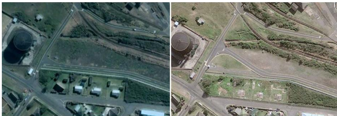
Figure 8.20. Consecutive Google Earth satellite images dated August 2004 (left) and August 2009 (right) showing the four houses on the proposed PV site, pre- and post-demolition (Source: Google earth).
