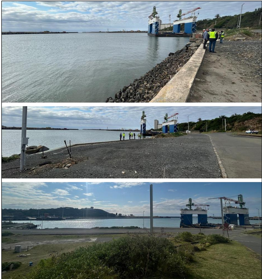
Figure 8.4. Views of the proposed estuarine intake and pump house site. Top and bottom: The proposed intake pipeline will protrude into the estuarine waters. Middel: The proposed pump house would be situated on the compacted dirt concrete surface.
