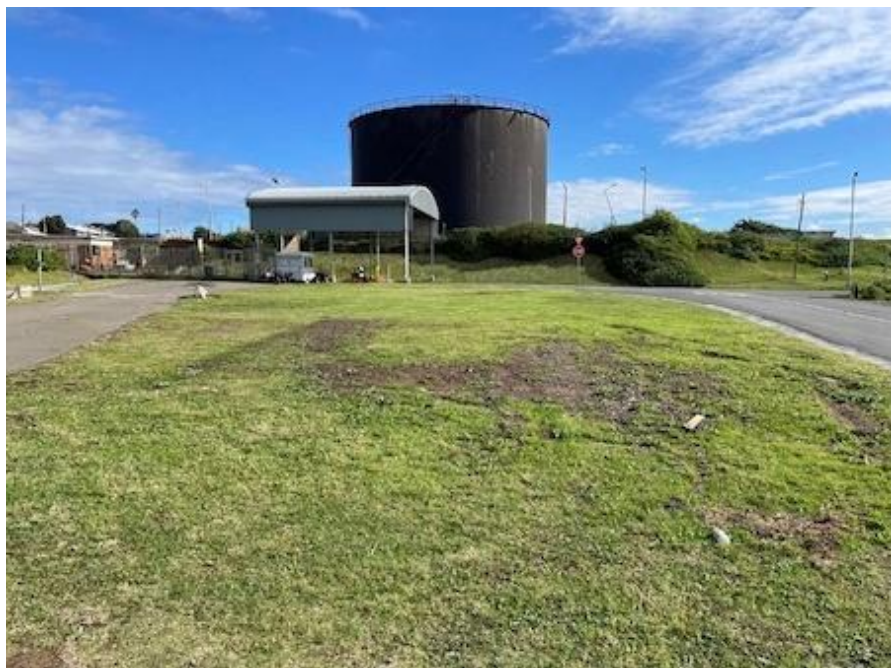
Figure 8.2. The proposed RO Plant site (grassed area) with the TNPA West Bank security entrance in the distance.
