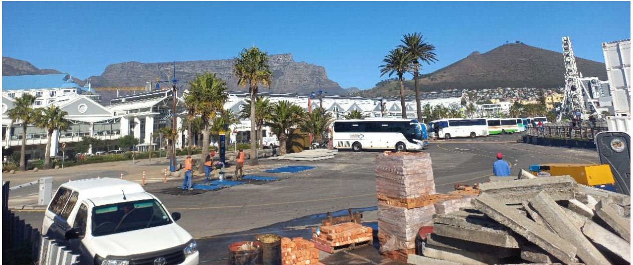
Figure 5. Parcel O, currently functioning as a roadway, parking area, and container storage. It is also used for temporary storage of construction materials.
