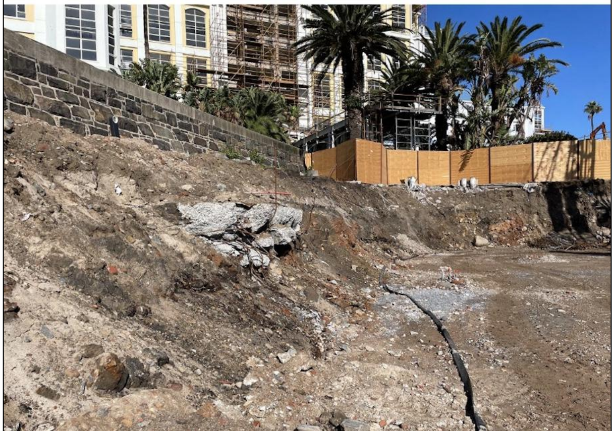
Plate 2: Views of the fill comprising the made ground, exposed during basement excavations in Portions Q and R of the Granger Bay precinct site adjacent to the proposed Phase 1B development site (Photos: J Kaplan).
