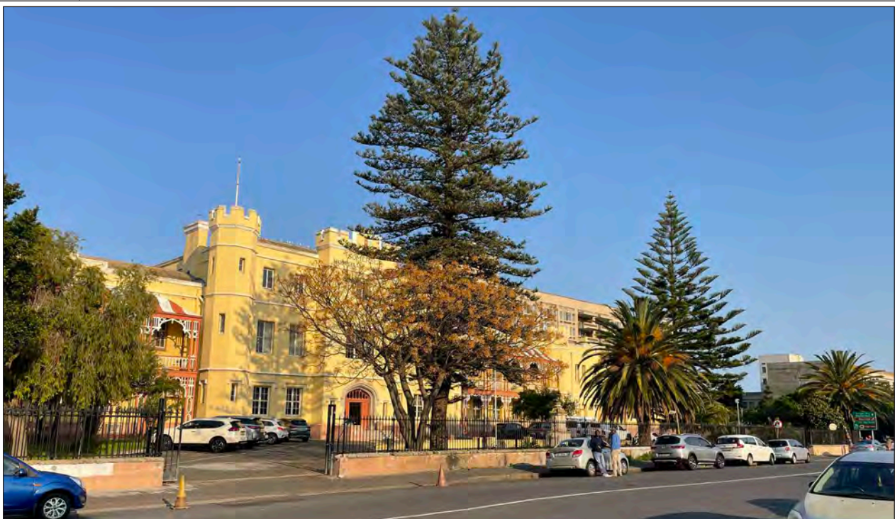
Figure 22E: Somerset Hospital is a stately landmark and a major organising townscape element for the precinct.
