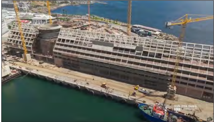
Figure 25C & D: Drone views of the Quay 7 building under construction clearly show that the structure creates a visual “viewshed” between the Victoria Basin and the site.
