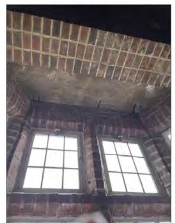
Figure 6H: Reinforced Concrete slab at Oriel.
