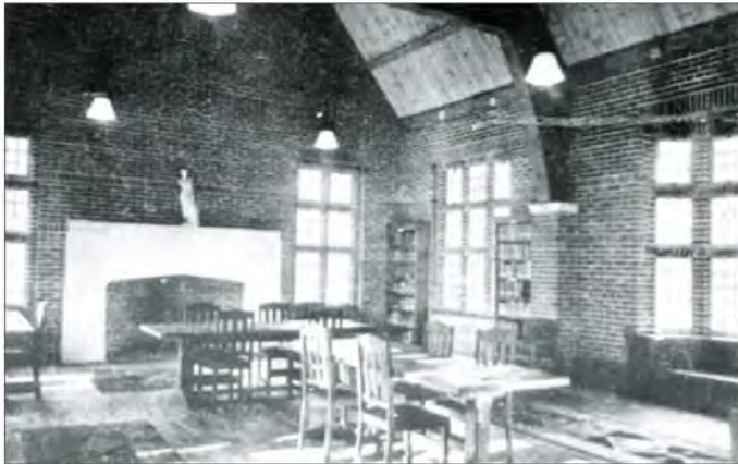
Figure 4B: The interior of the space when it was being used as a library - the initial purpose of the structure - taken c1940. (Old Herschillian News, Archives and Heritage).
