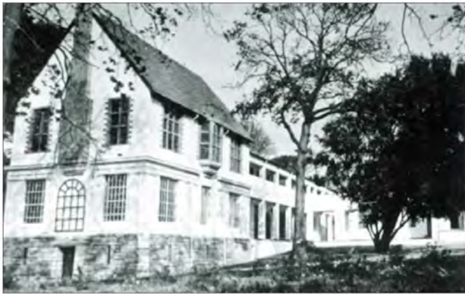
Figure 4A: The northern gable end of the building, taken c1940. (Old Herschillian News, Archives and Heritage).
