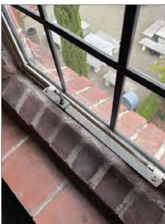
Figure 6E: View of the chaped cill bricks.
