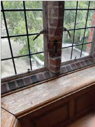
Figure 6A: Spawling mullion in Oriel window.
