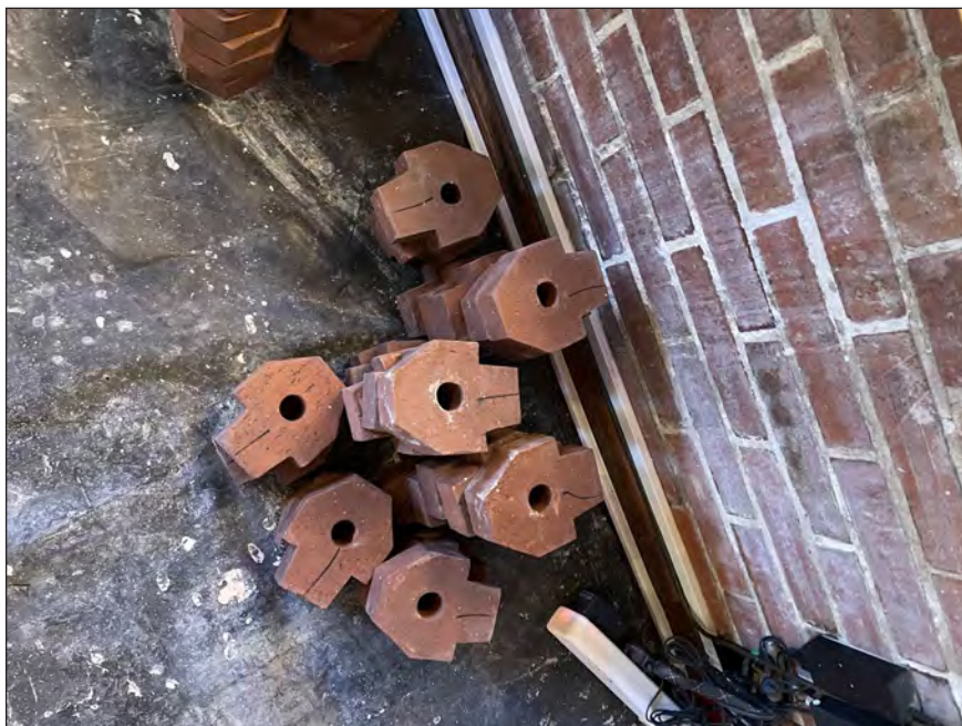
Photographs from the on-site monitoring, showing the reconstructed windows, with the custom-manufactured bricks that had to be used in the reconstruction.
