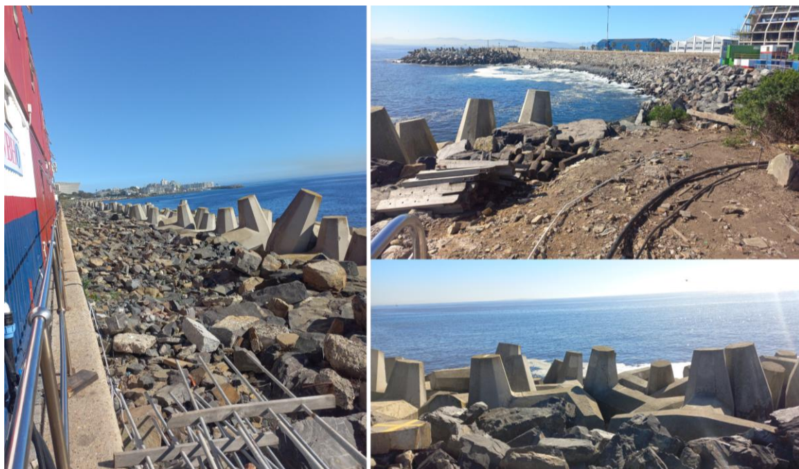
Figure 5. The shoreline protection and retaining wall separating the development site from the marine environment (photos from May 2025 site visit).
