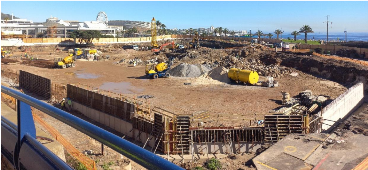
Figure 4.8. Construction of another development occurring south of the proposed site. Parcel P is located to the right of the construction area (not fully visible in this photo), while Parcels O and a1 & a2 are visible in the distance near the grass and palm trees.
