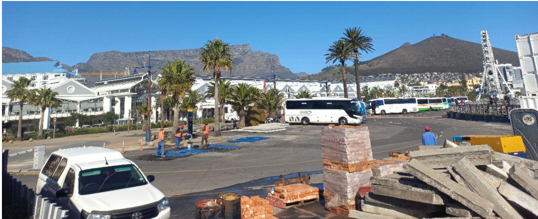
Figure 4.12 Parcel O, currently functioning as a roadway, parking area, and container storage. It is also used for temporary storage of construction materials.
