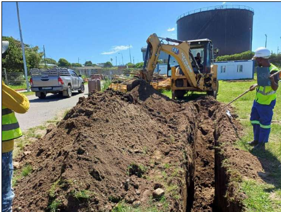
Photo 1: Test pit excavation on DS 3
