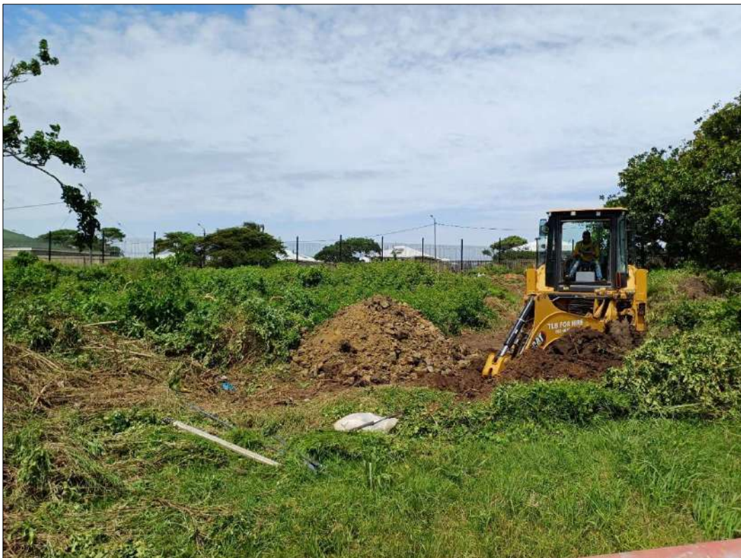
Photo 2: Test pit excavation on the Reservoir position
