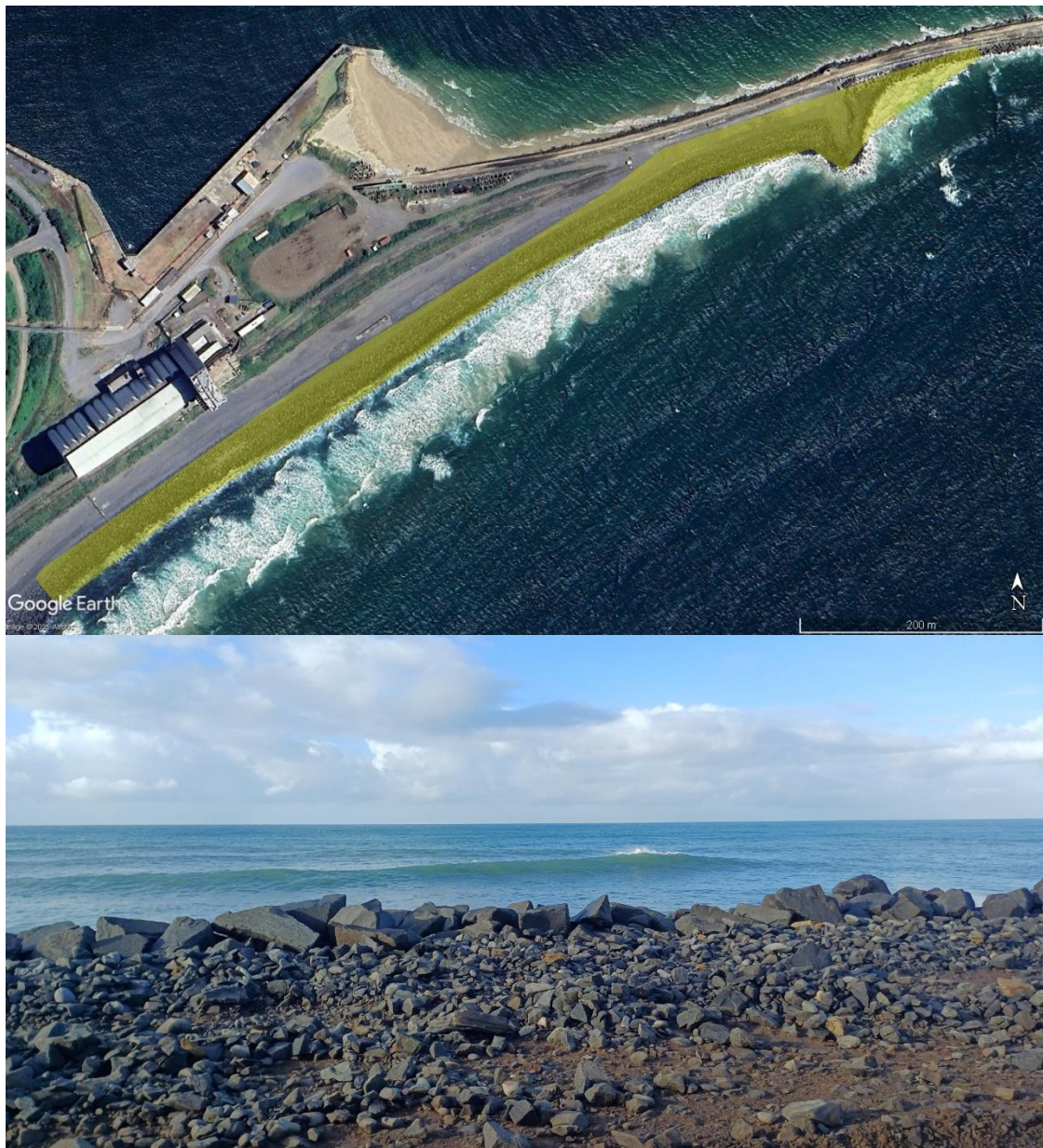
Figure 3.4. The beach to the south of the Port of East London entrance is comprised almost entirely of artificial dolosse habitat.
