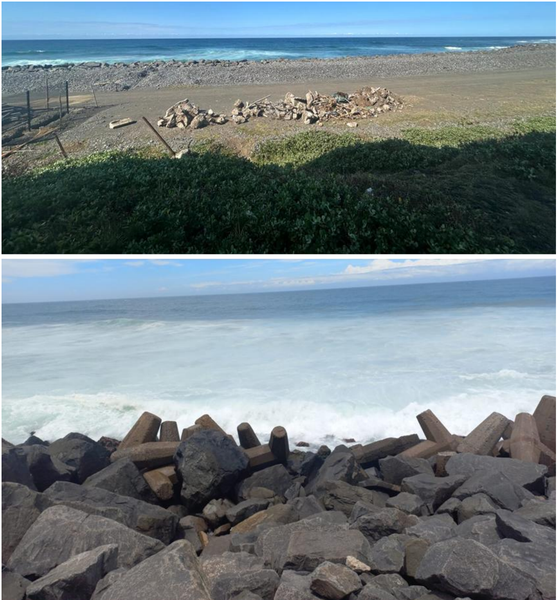
Figure 8.5. Site photographs captured in 2025. Top: View looking east towards the ocean, showing the service road, rocky shoreline, and dolosse at the water's edge. Bottom: Closer view of the breakwater comprising rock armour and dolosse, across which the pipeline will be routed and at which it will terminate.
