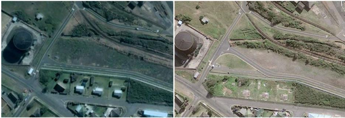
Figure 8.22. Consecutive Google Earth satellite images dated August 2004 (left) and August 2009 (right) showing the four houses on the proposed PV site, pre- and post-demolition (Source: Google earth).
